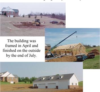
Next came wiring, plumbing, insulation and drywall. We painted the interior in November and had the hoist installed in May 2004.
